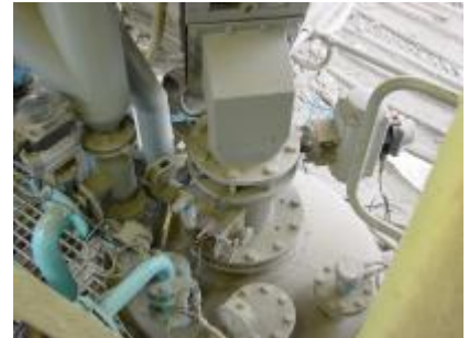
Cone Filling Valve on cement batching plant ▼
