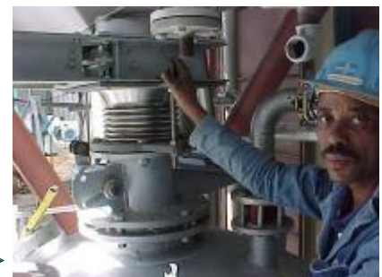
Pressure Vessel filling arrangement: Knife Gate, Compensator with Cone Valve →
