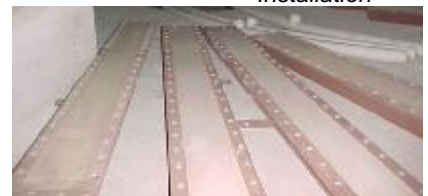
Typical Silo Aeration Pad Installation
