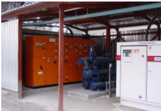
Electrical System Upgrade
