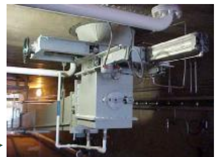
Silo Discharge Arrangement - Manual Knife Gate valve with Pneumatic Knife Gate Valve combination in an Aeroslide system
