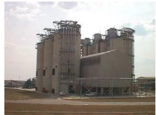
Ash storage silo with pneumatic conveying piping and dust suppression filters
